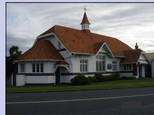
Musselburgh Church Queens Drive
